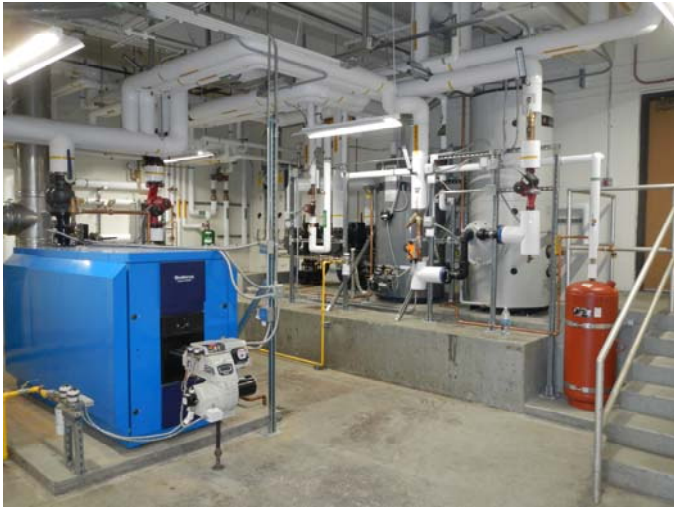
Kodiak Middle School Boiler Room Remodel
