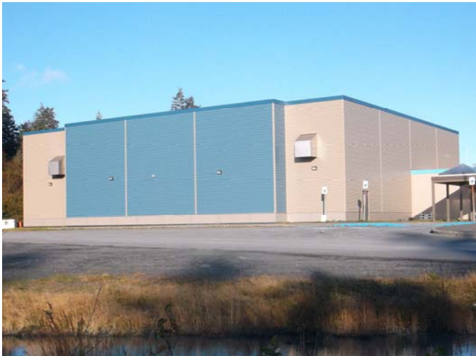
North Star Elementary Gym Siding
