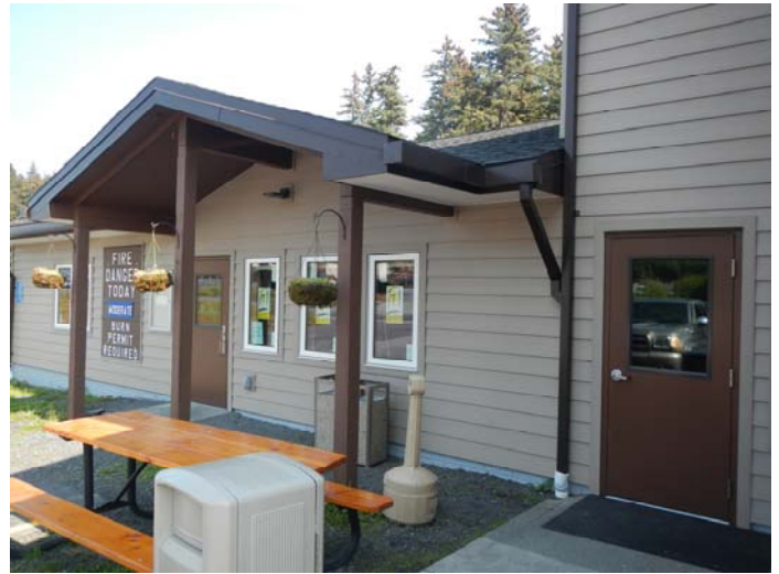
Bayside Fire Department Exterior Improvements
